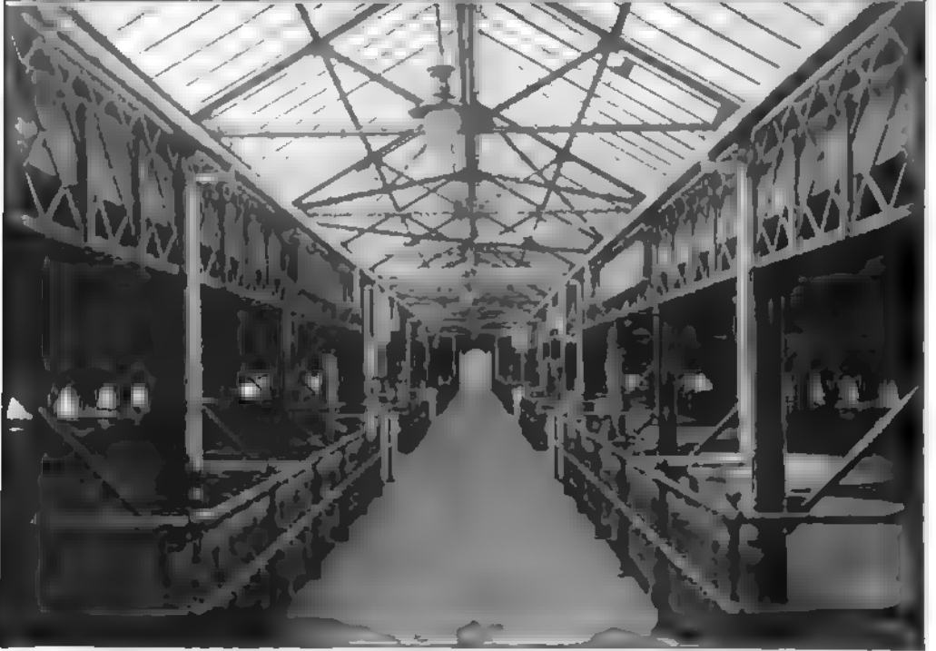
1 Toronto Drifting Sand Filters (view from south west) 2 Toronto Drifting Sand Filters — Filter Gallery and Filters (looking north)
